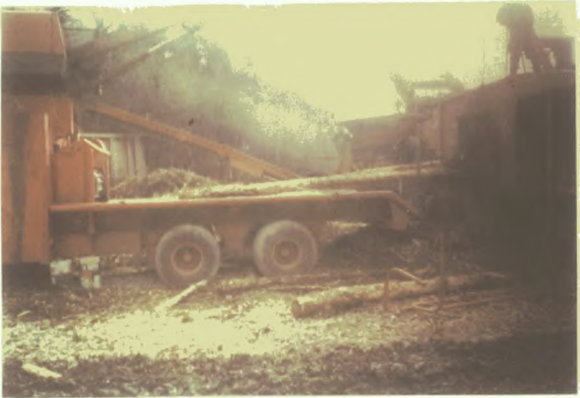
Plate No. 5 : This illustration shows clean stems emerging from the Mantowoc. The stems are being grabbed by the grapple of the Morbark chipper and are about to be fed in through the steel feeding roller which can be seen to the left of the stems.
