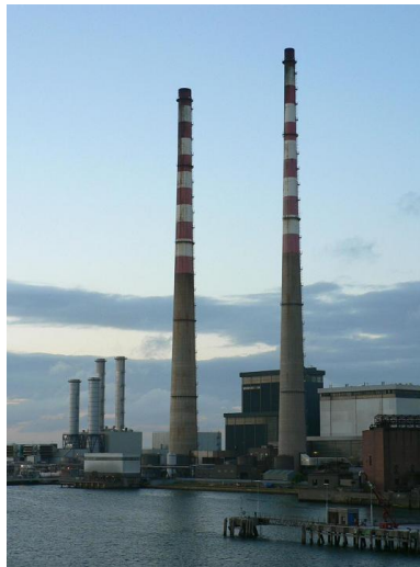
Figure 2 Poolbeg fossil fuel power station Ireland [4].
