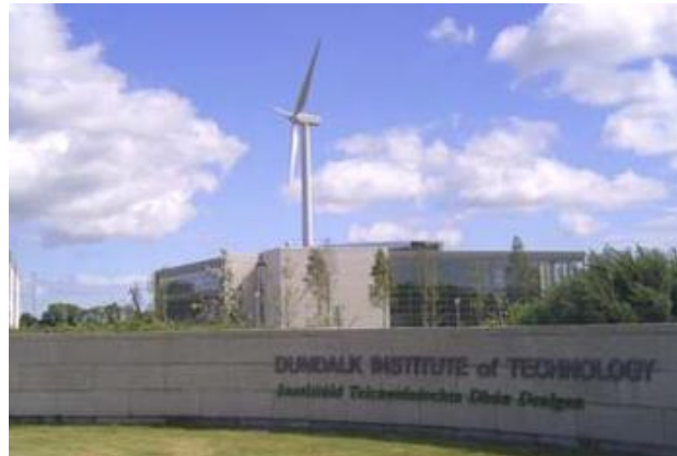
Figure 8 Wind turbine at the Dundalk institute of technology.
