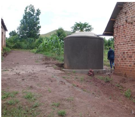
Figure 2.9 Harvested rainwater tank used to supply water to the PMMA reactors in Uganda
