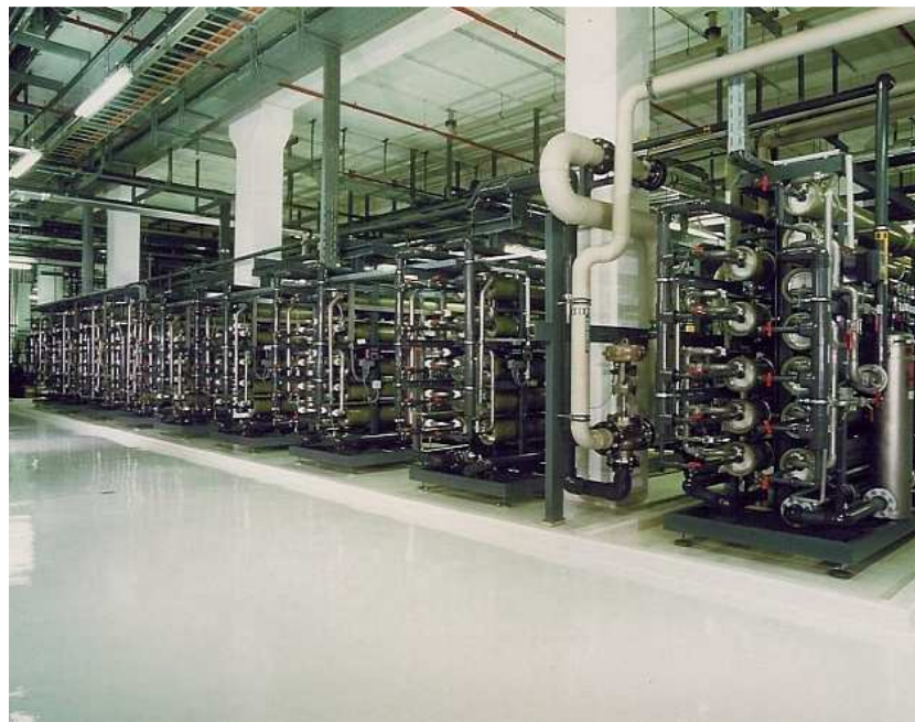
Figure 2-6: RO arrays in a UPW plant [53]
