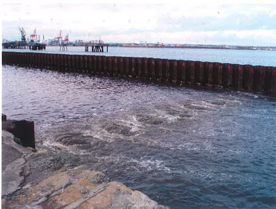
Plate 2.14: Point of discharge of the WWTP effluent into the cooling water flowing from ESB power station, and thence into the water of Dublin Bay
