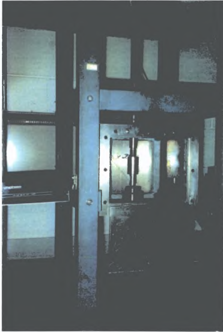
Plate 4.4 Shows view of the Shield Box.
