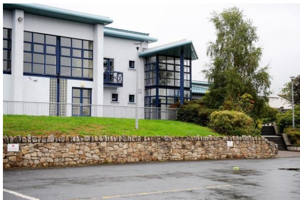
Figure 3.13. Ballyway Secondary School
