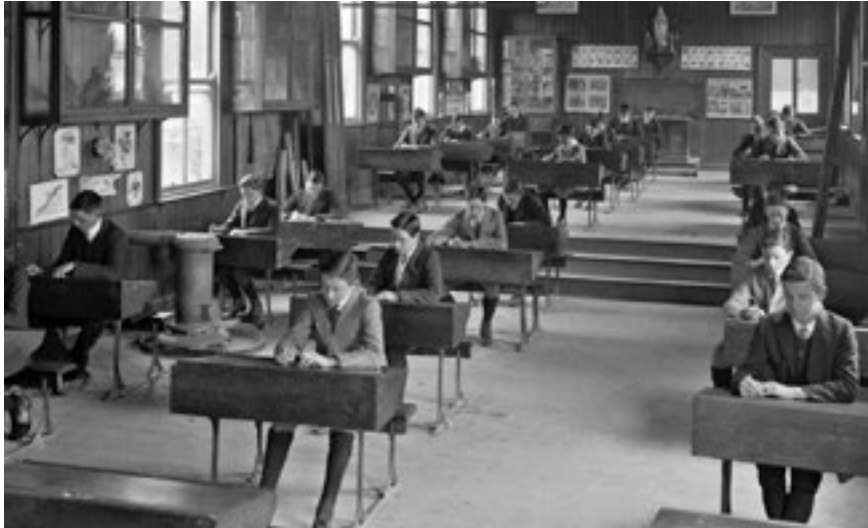
Classroom in Waterpark College, Waterford.
