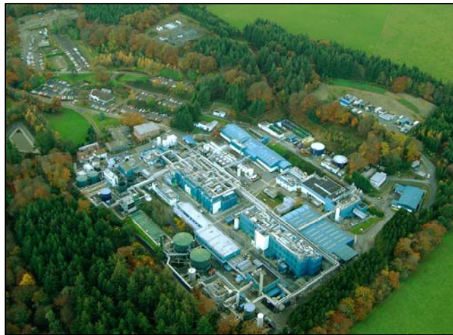
Fig.8. Aerial overview of Schering-Plough (Avondale) Co.
